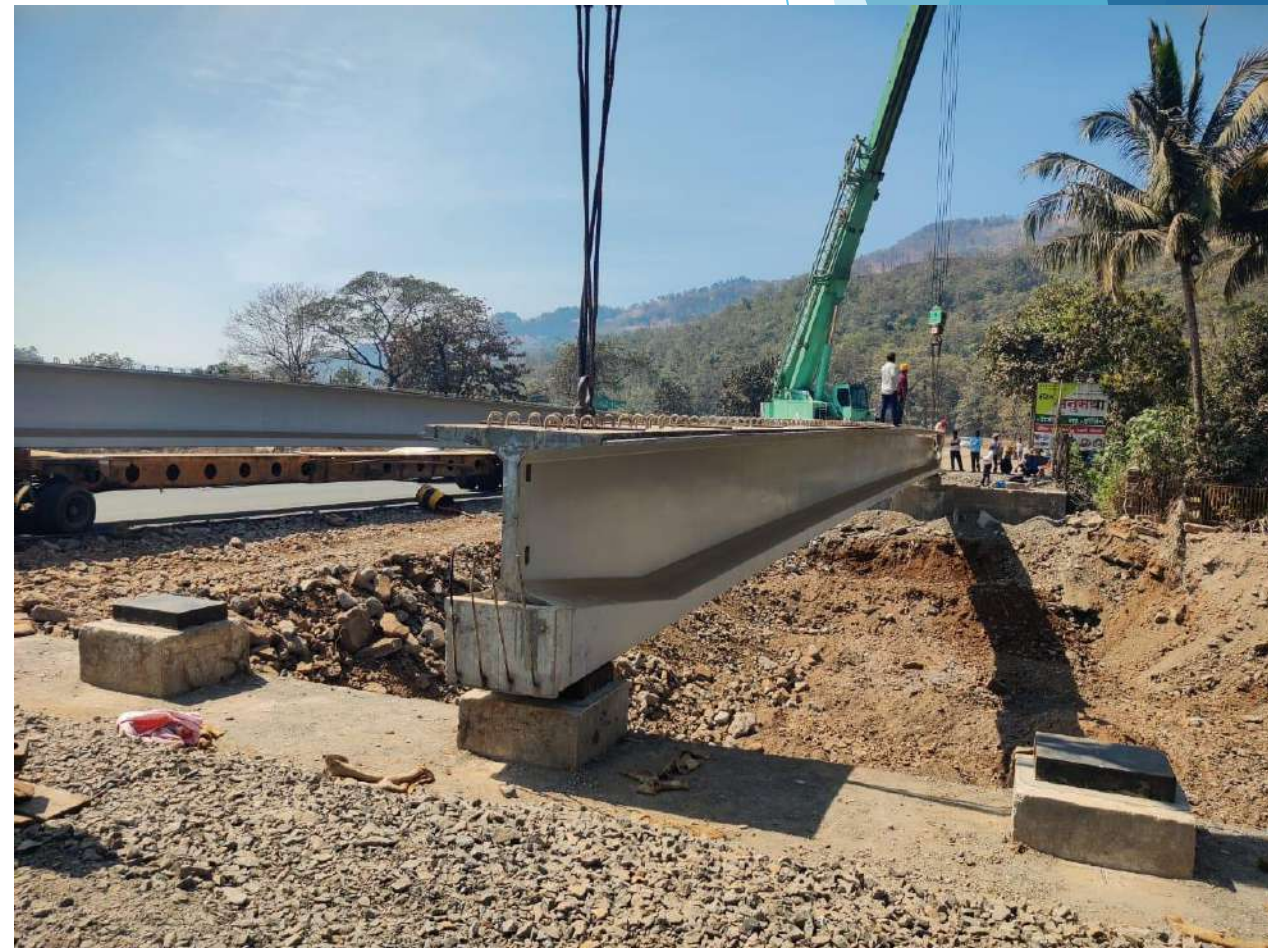
Erection Works in Progress at Kashedi Ghat Project
