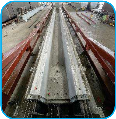
Release of Pre-tensioning
