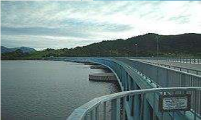
The Bergsøysund Bridge
