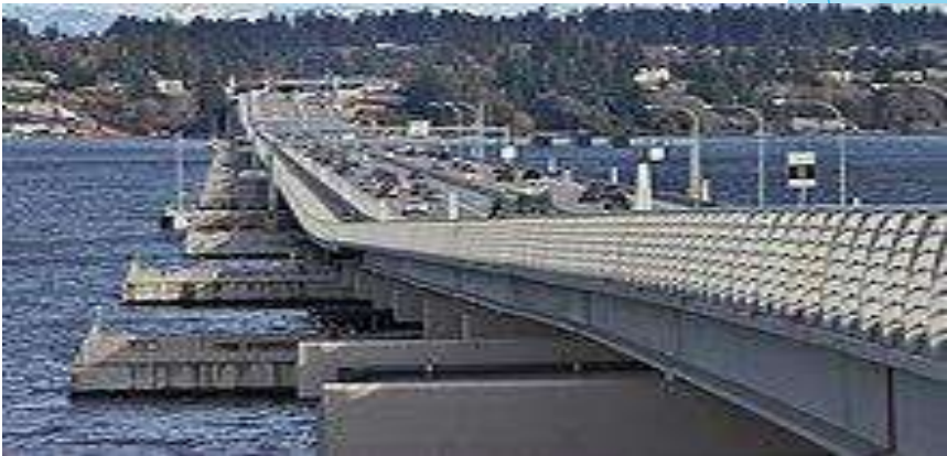
The Evergreen Point Floating Bridge
