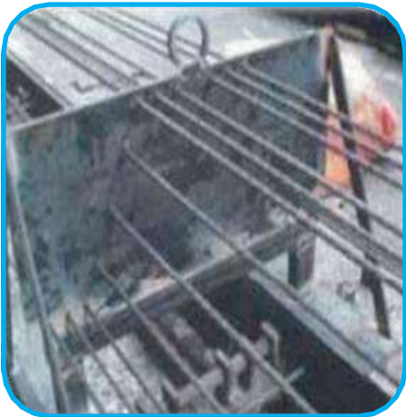
Placing and Prestressing
