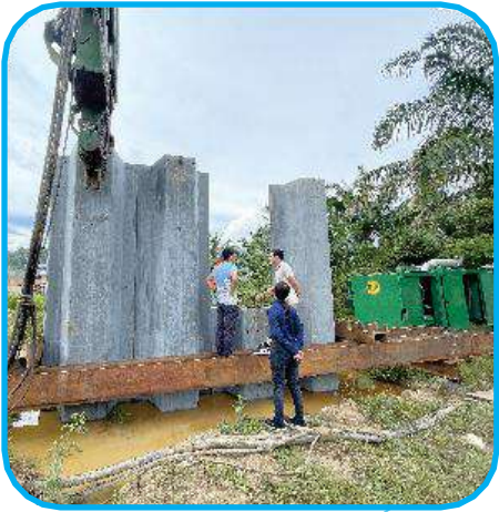
Driving of sheet pile
