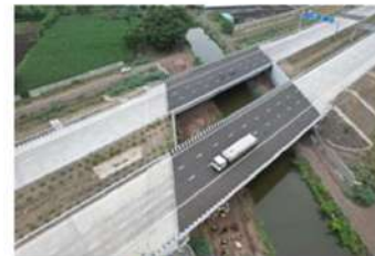
ROB over canal Samruddhi Expressway
