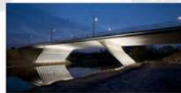
Republique bridge (France) - 2017
