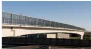
Sherbrooke footbridge (Canada) - 1997
