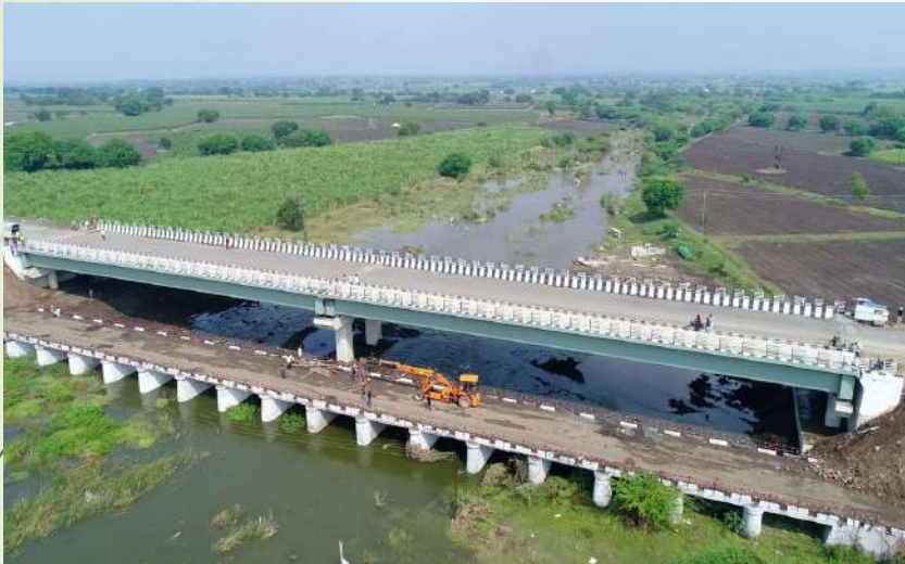
Bridge at Latur May 2021
