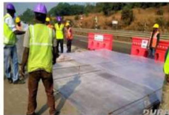
Pavement overlay Mumbai – Pune Expressway
