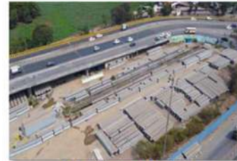
Rehabilitation of Bridge Turbhe
