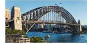
Harbour railway bridge deck upgrade (Australia) - 2022
