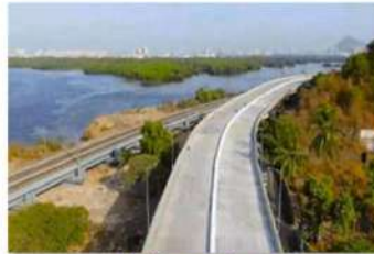
Bridge overlay Mumbra
