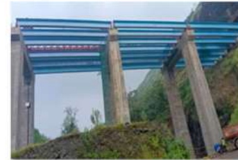
Viaducts Pune Mumbai Expressway (Missing link)
