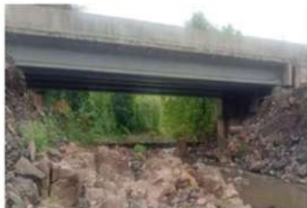
ROB over canal Panvel Mahad – Panjim road
