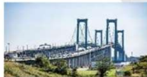
Delaware memorial bridge deck overlay (USA)- 2023
