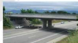
Bourg-lès-Valence bridge (France) - 2002
