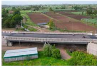
Lane extension of 2-lane stretch Dharampuri
